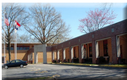
The City Center opened its doors on May 8, 1993 to coincide with Shrewsbury's 80th year of incorporation
