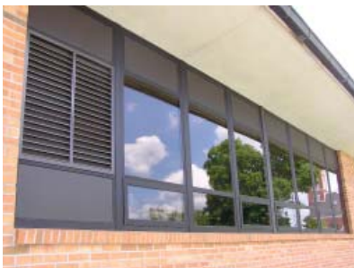
New Windows / Heat Pump Louvers
