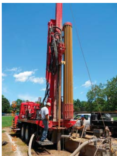
Geothermal Well Drilling
