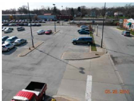
The geothermal system well field is located under this section of the parking lot. The field has 24 wells that are 400 ft. deep.
