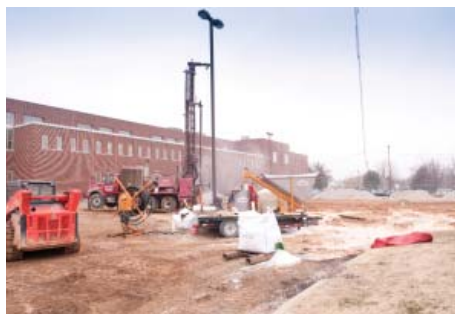
Well Field Drilling. The field is comprised of 54 wells drilled 330 feet deep.
